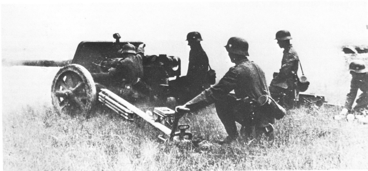
ABOVE: A rare photograph of a 7.5 cm Pak 41 in action. Only 150 units of this tapered bore Gerlich system gun were built. Note the periscopic sight. This Krupp design had a taper bore, 7.5 cm at the breech, reducing to 5.5 cm at the muzzle end. The bore was prone to wear and tungsten cored ammunition was not available in large enough quantities were two factors which reduced the chances of this gun being adopted for production. Its competitor the 7.5 cm Pak 40 was produced instead.
